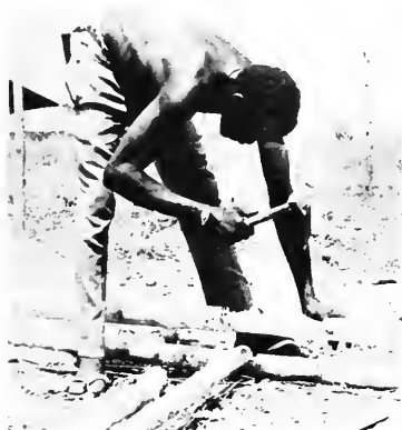
Erecting center for refugees, Sudan
